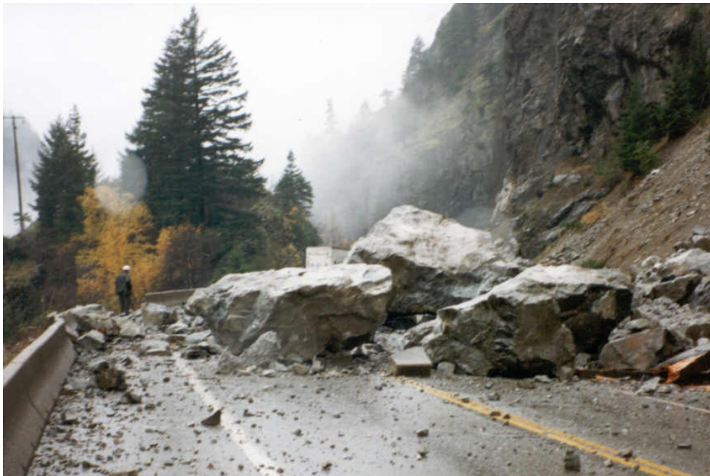
Figure 1 – Rock fall from hazardous slope, with high risk to highway because of minimal catch ditch and short pathway.
